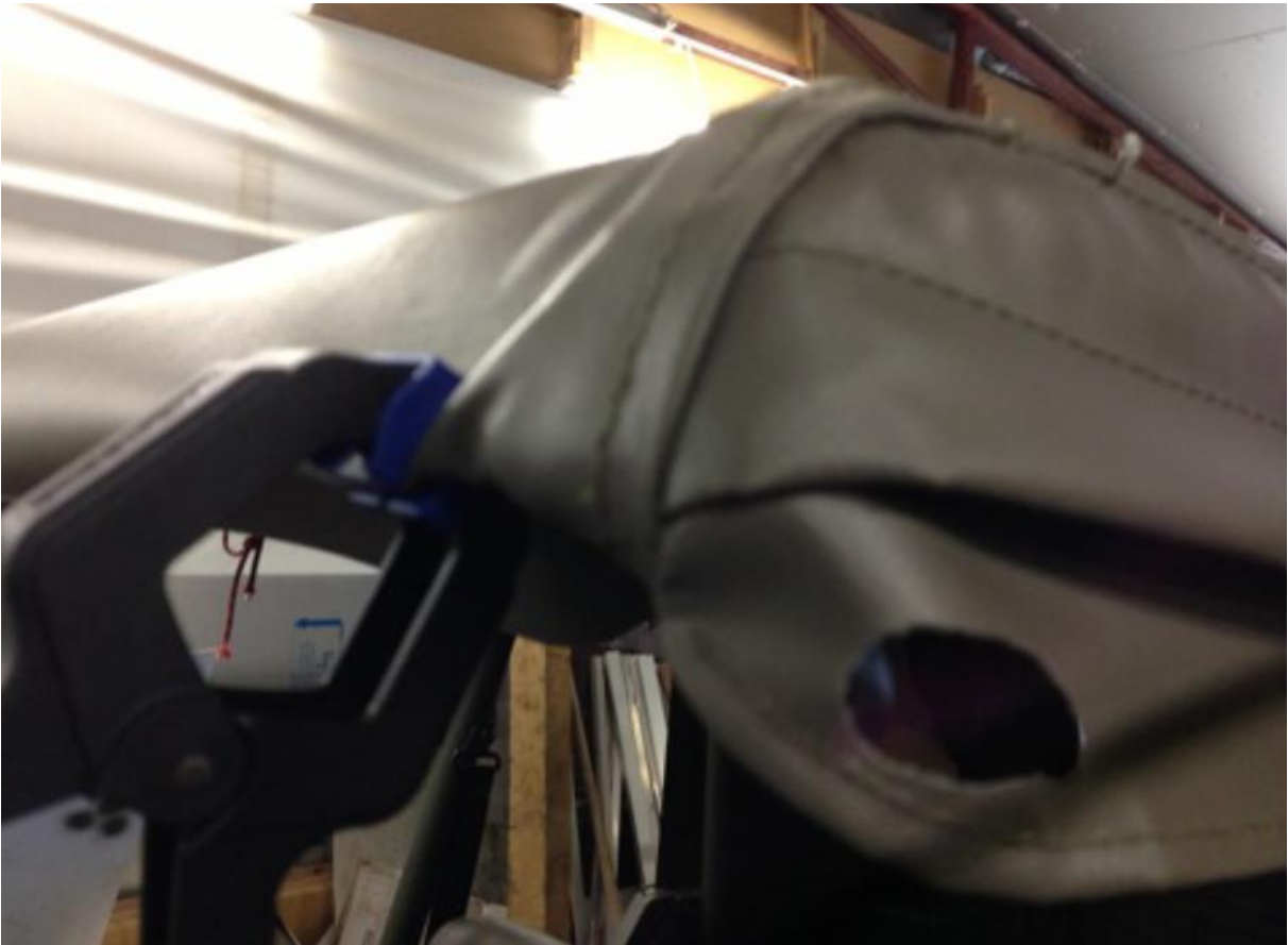
The tarpaulin is now fixed with clamps at at least 3 points.
